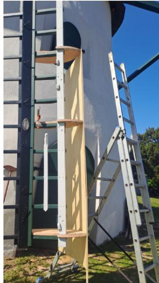
*The leading edge glued and nailed to the three formers.*
