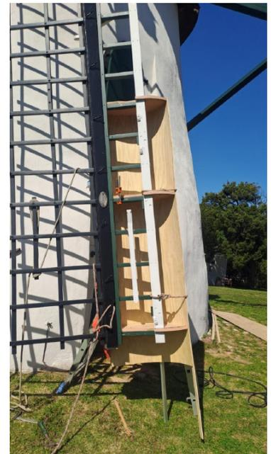
*Top and bottom trimmed off and cover-strips attached.*
