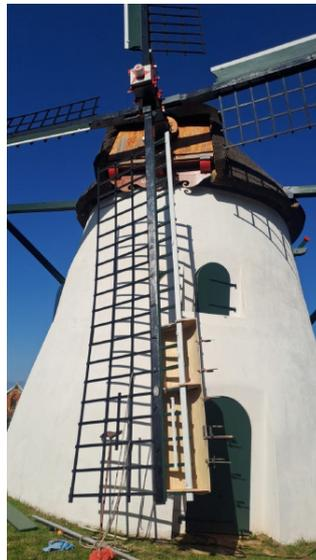
I took it home and tidied it up and gave it coats of pink primer and universal undercoat. On the next visit, we tested it. It slipped over easily but we found it difficult to align the bolt holes exactly, so we removed the captive nuts and drilled 9mm holes for the 8mm bolts and used longer bolts and wing nuts. We left it on while we worked on the second jib.
