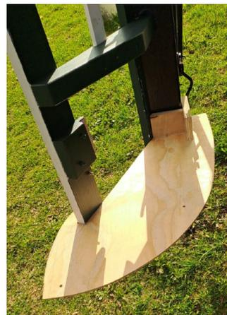
*Testing the first pattern on the outer sail bar on stock No 2, an outer.*
