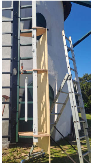
Using ropes to pull the ply against the formers.
