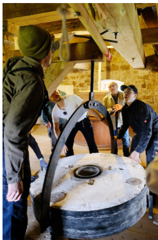
Gerrit, Björn and Johann lift the runner stone at Exter Windmill using the millstone crane.
