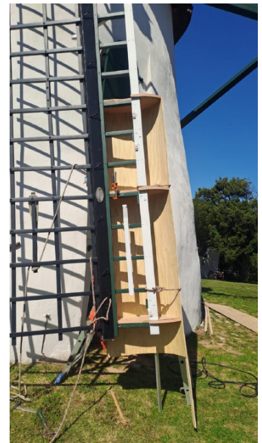
Using ropes to pull the ply against the formers.
