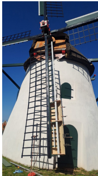
Top and bottom trimmed off and cover-strips attached.
