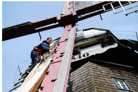
Johann climbs up the sail of the Feldmühle in Martfeld, to fix the cloth.
