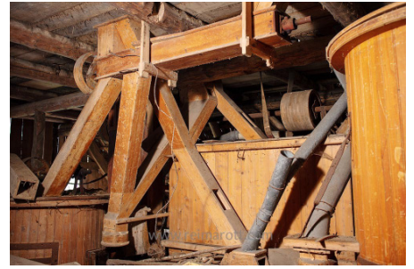
The roller mill in Steinbeck Mill is standing still for more than 40 years.
